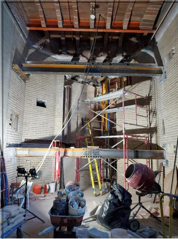
To allow for the insertion of the new elevator and stair, three floors of the Coxe Wing were removed and required a complex construction sequence. In this area, original windows and skylights were also reopened to bring in daylight.
